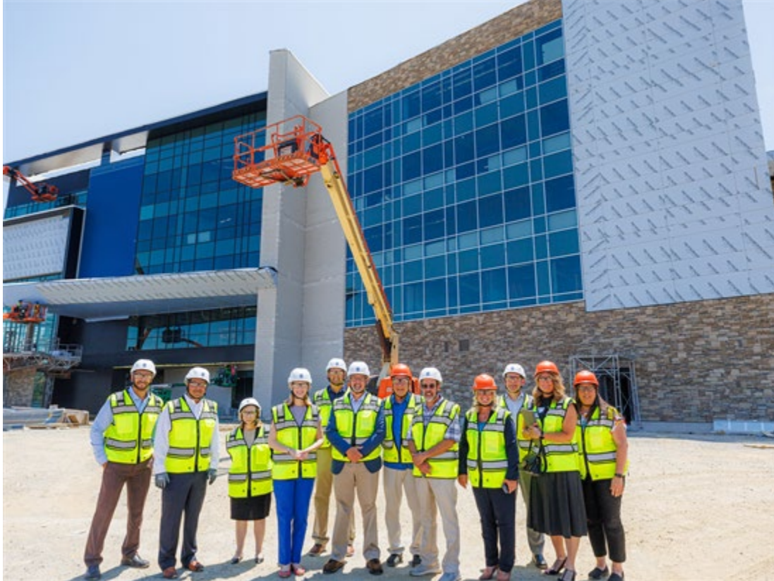
Comptroller Lierman dons a hard hat at the construction site for the School of Medicine at Meritus Health in Hagerstown on Friday, June 21, 2024.
