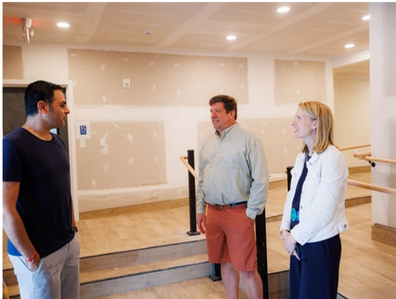
Comptroller Brooke Lierman tours Phillips Crab House housing renovation with developer Mike Ramadan (left) and Delegate Wayne Harman
